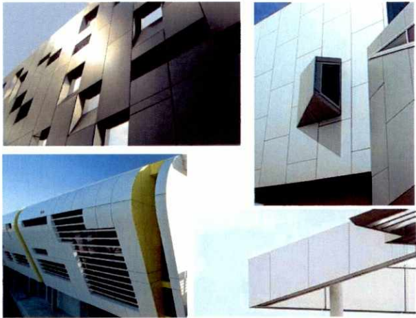
FSC - EXAMPLES OF FRAMED SHEET CLADDING PANELS
